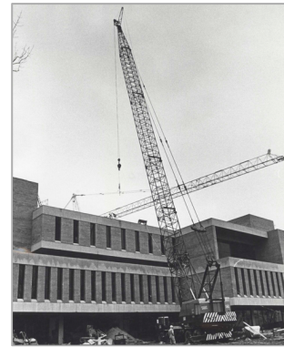
Wyllie Hall under construction
