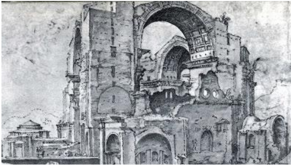
St. Peter's Under Construction, 16 th Century
